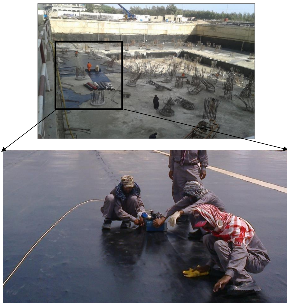
Figure 6.2: Highrise basement water proofing with PVC geomembrane
